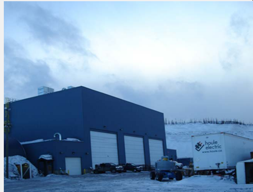
Maintenance and Warehouse Building
