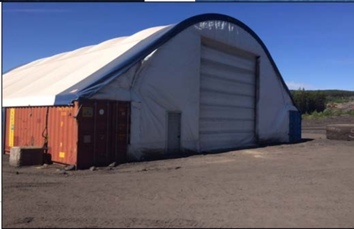
Tire Shop and Light Vehicle Shop
