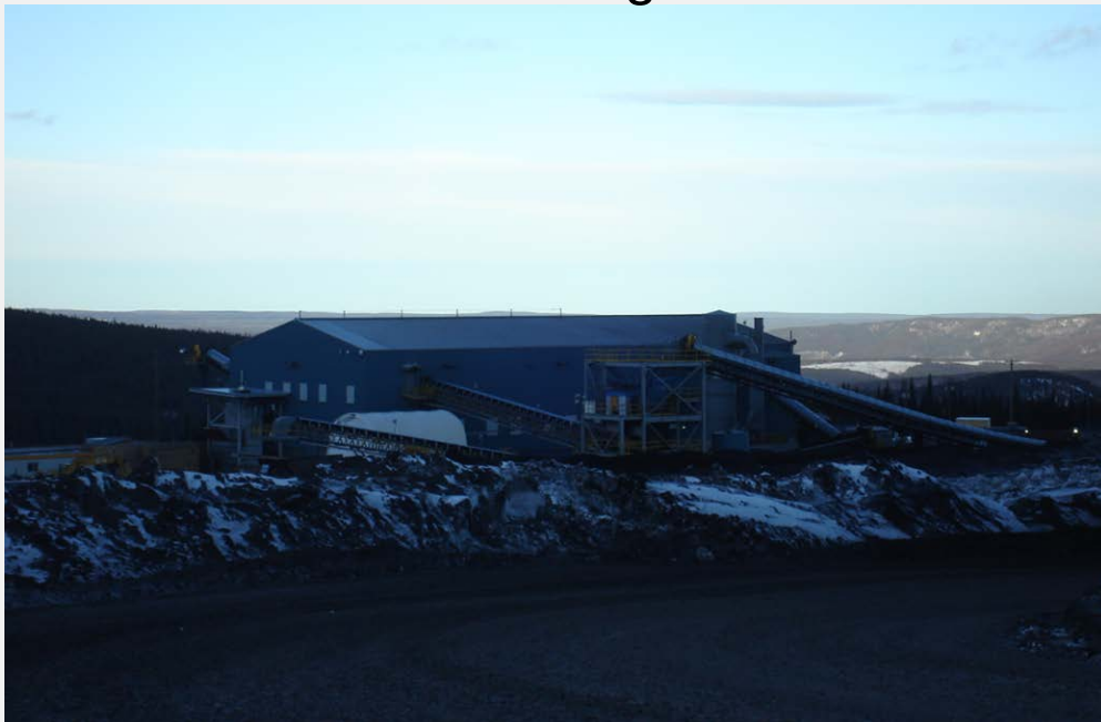
Coal Processing Plant
