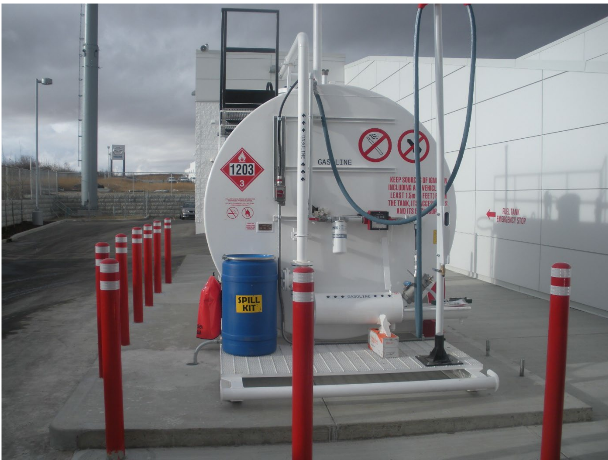
Figure 1.18-3: Example of Light Vehicle Fueling Station
