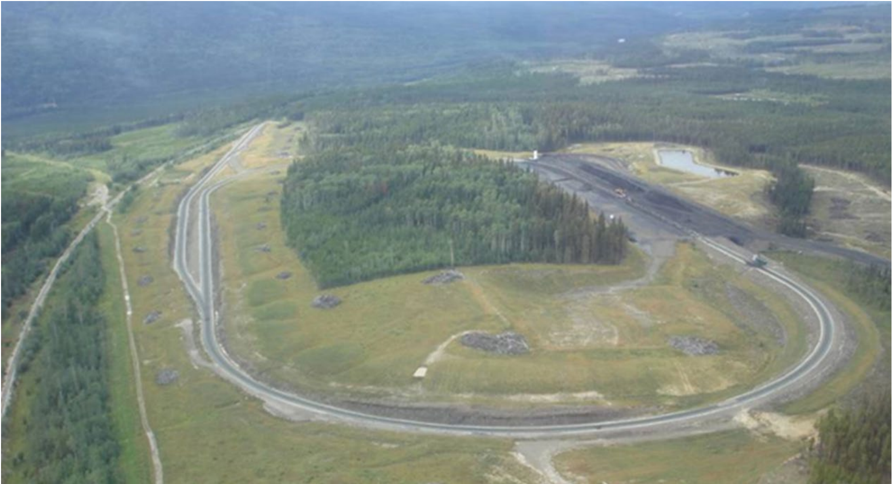
Figure 1.21-2: Photo of similar Rail Infrastructure design for the Project
