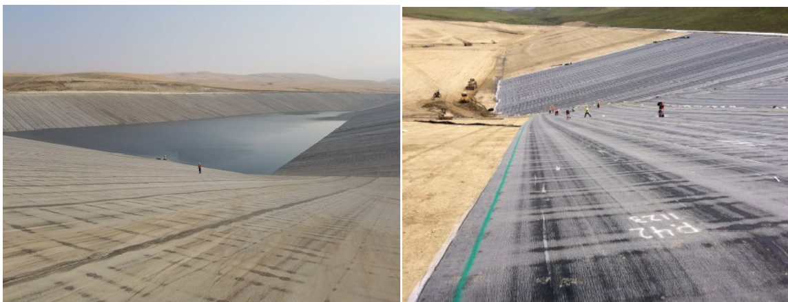
Figure 1.22-19: Typical installation of a bituminous liner in a large sedimentation pond
