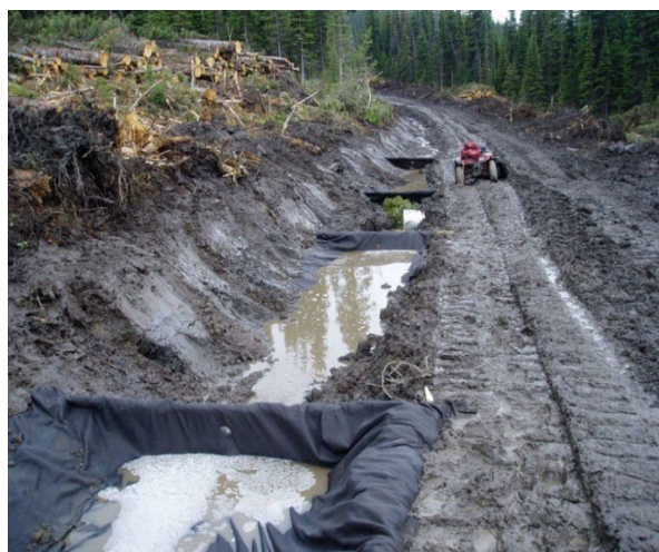
Figure 6.6-5: Examples of temporary erosion and sediment control methods
