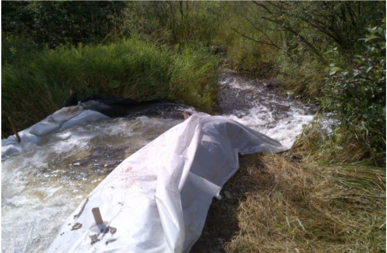
Figure 6.6-4: Passive diversion technique – temporary poly-lined channel
