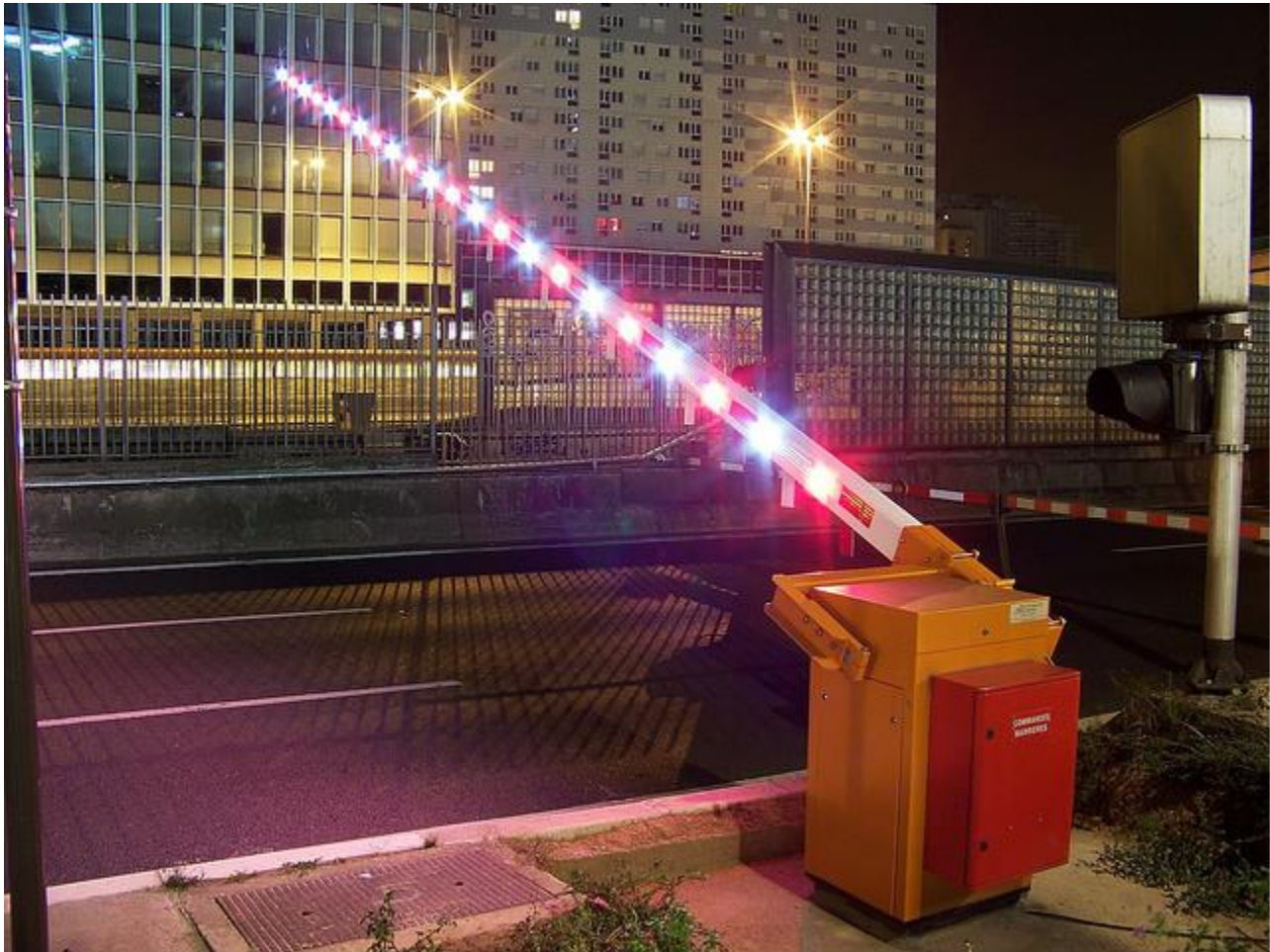
Figure 6.5-1: Example of an access control gate
