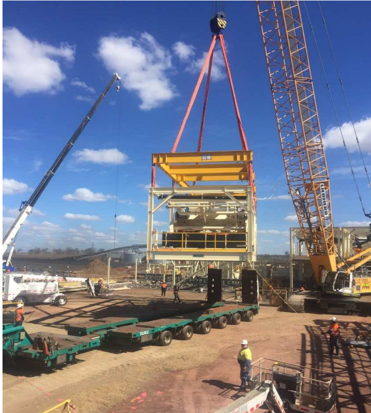
Figure 6-4 Crane lifting module for installation
