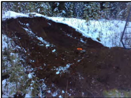
Photo 1: Test pit excavation.
