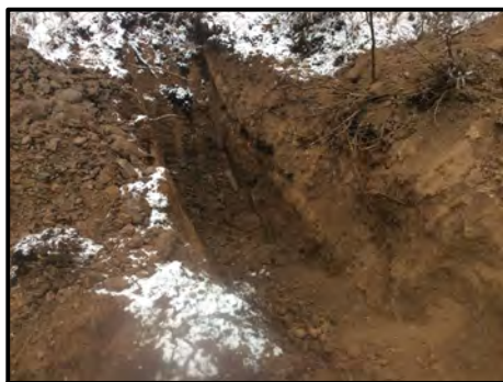
Photo 1: Test pit excavation.
