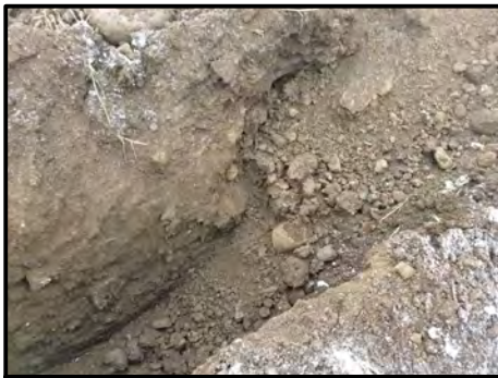
Photo 1: Test pit excavation.
