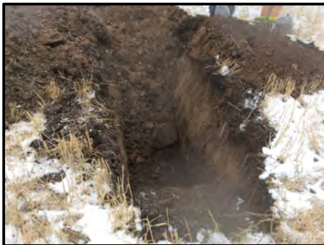
Photo 1: Test pit excavation.
