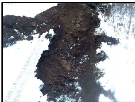
Photo 1: Test pit excavation.
