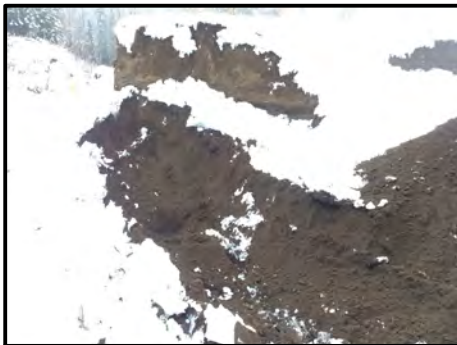
Photo 1: Test pit excavation.
