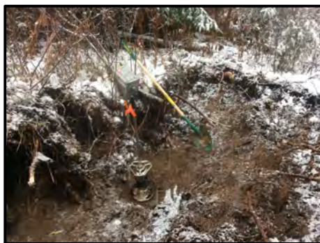
Photo 1: Test pit excavation.
