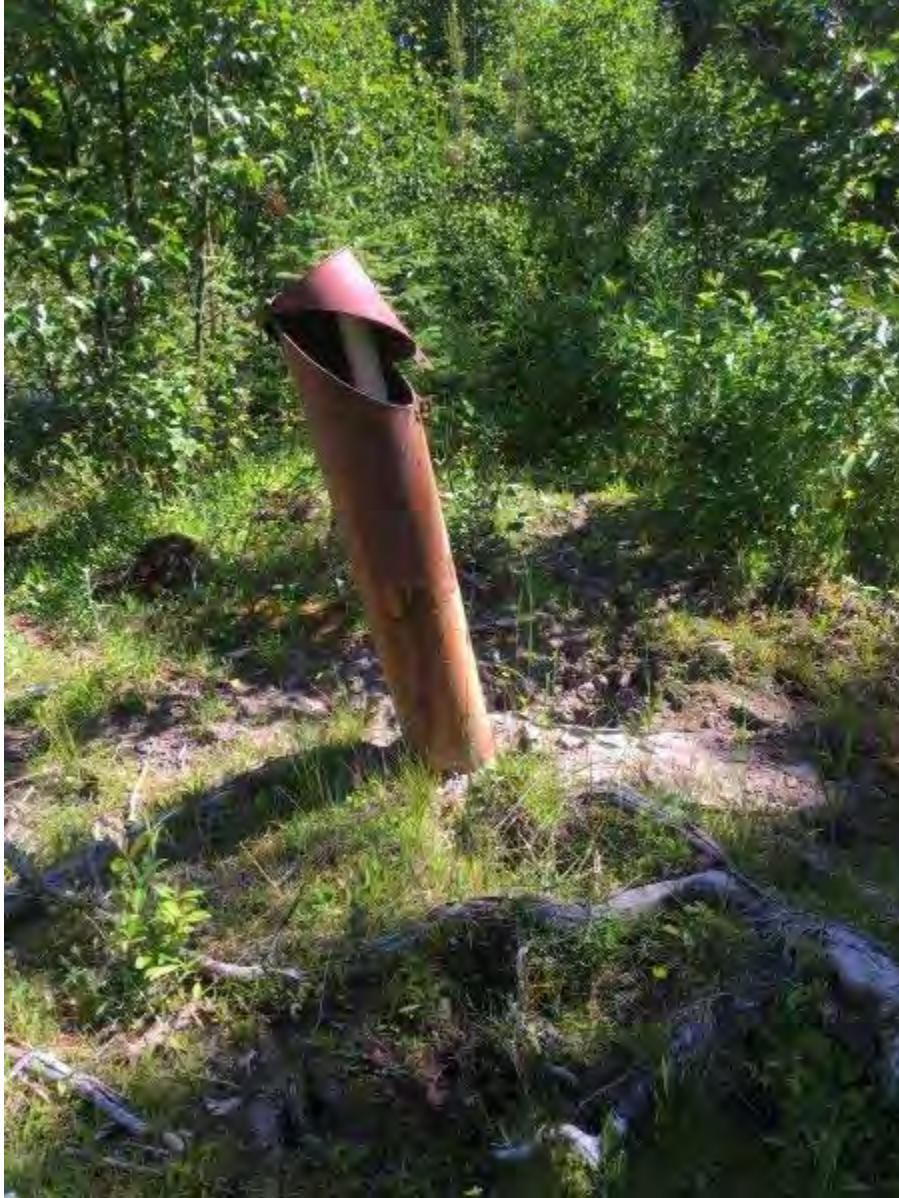
Photo 1 - Damaged Well T96R-56C-83
