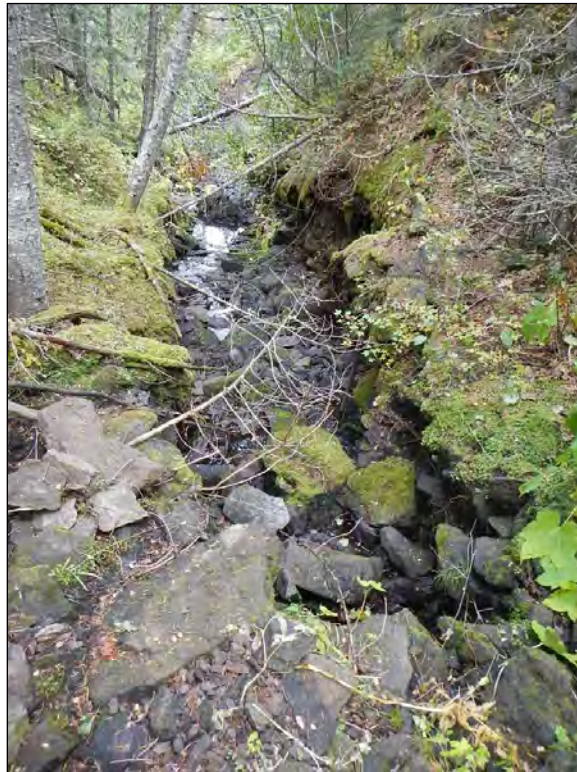
Photo 11.5-13. East Fork Tenas Creek tributary, looking downstream through the steep, dewatered canyon section. October 9, 2018.
