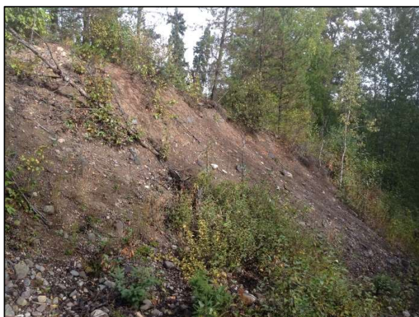
Plate 2-9. Road cut in sandy gravel above the Telkwa River, field site IW133.
