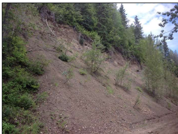
Plate 2-1: Bedrock cliff and ravelling colluvial slope along the Caribou FSR, fieldsite IW122.
