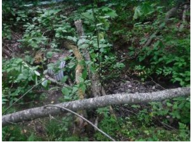
Photo 24. Inlet habitat at 900 mm culvert.
