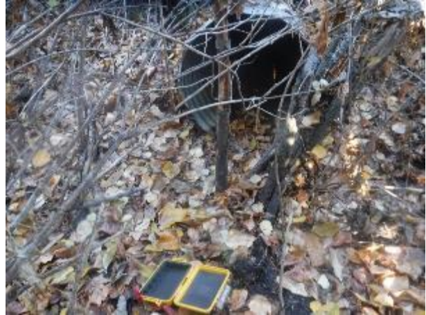
Photo 67: Upslope side of 600 mm culvert.
