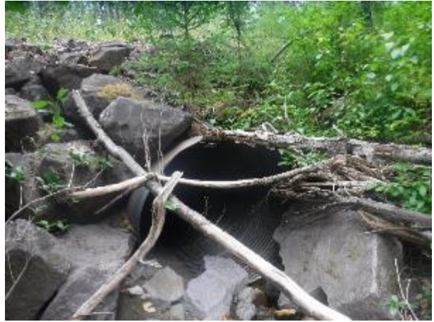
Photo 40. Upstream view of 1800 mm culvert.
