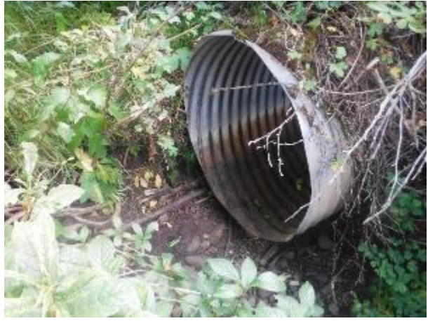
Photo 14. 900 mm culvert downstream of the proposed crossing.
