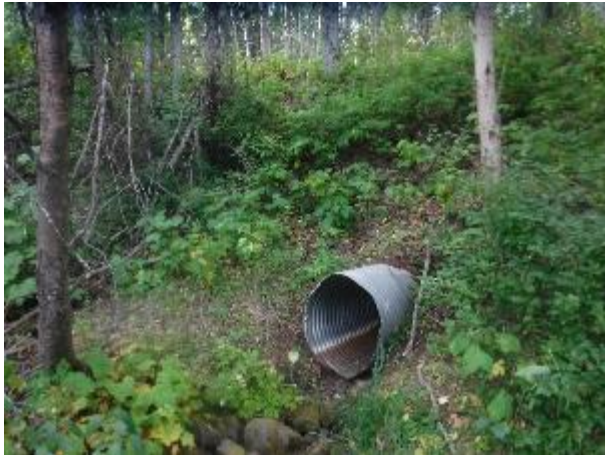
Photo 19. Downstream view of 900 mm culvert with small plunge pool and cobbles.
