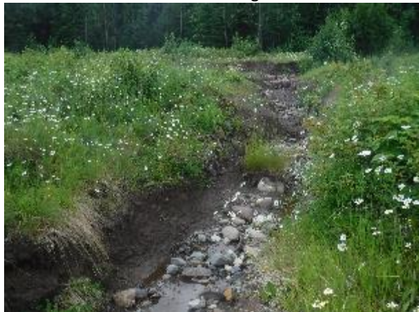
Photo 18. Well scoured reach (July 2020).
