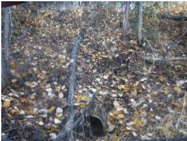
Photo 63: Crossing with functional 700 mm culvert and roughly 2.5-3 m of gravel fill.
