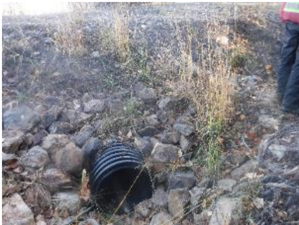
Photo 59: Newer, functional 500 mm culvert at crossing with a 1 m fill.
