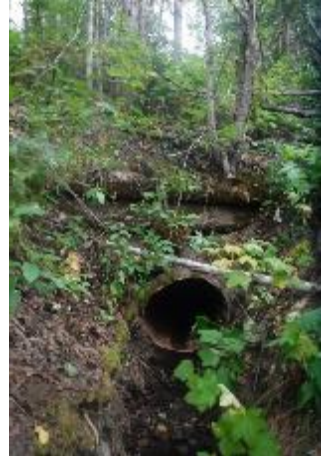
Photo 28. Outlet of 900 mm culvert at proposed road crossing.
