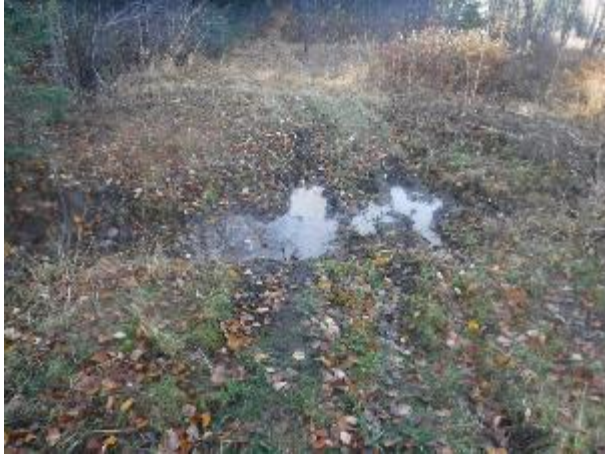
Photo 49: Crossditch at road crossing.
