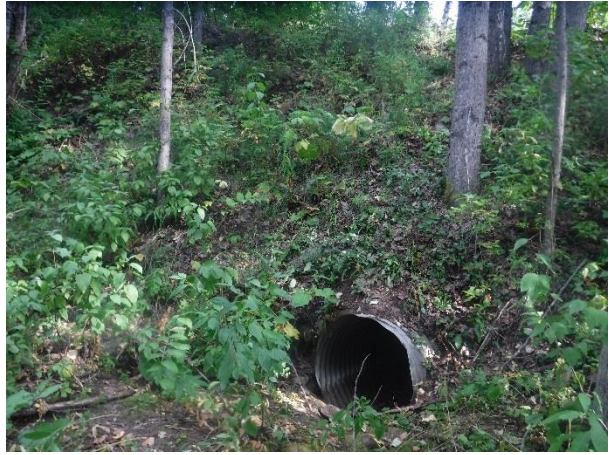
Photo 20. Upstream view of 900 mm culvert with overhanging vegetation present as cover.
