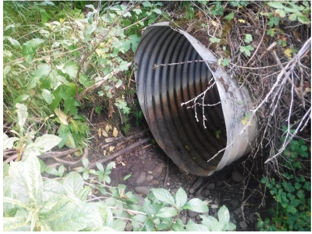
Photo 14. 900 mm culvert downstream of the proposed crossing.
