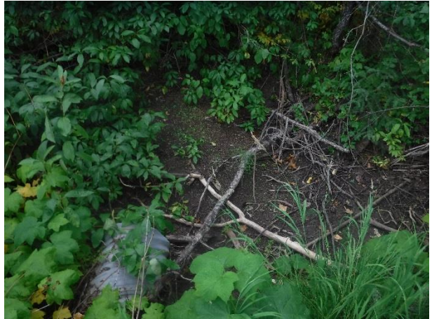
Photo 36. Upstream view of 500 mm culvert. Abundant fines.
