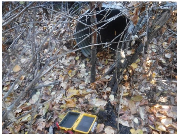
Photo 68: Upslope side of 600 mm culvert.
