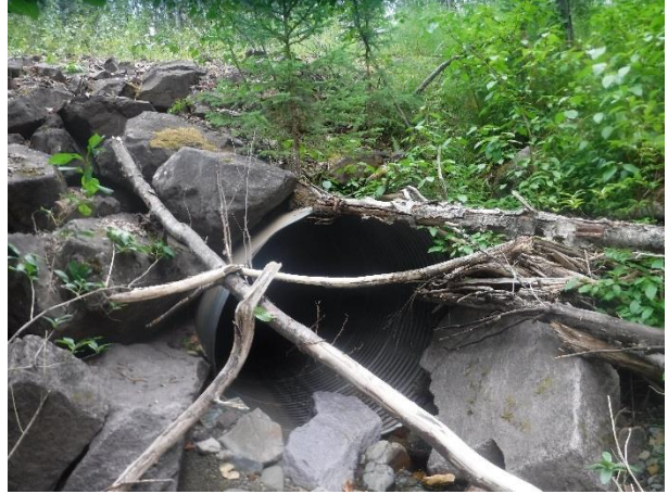
Photo 40. Upstream view of 1800 mm culvert.
