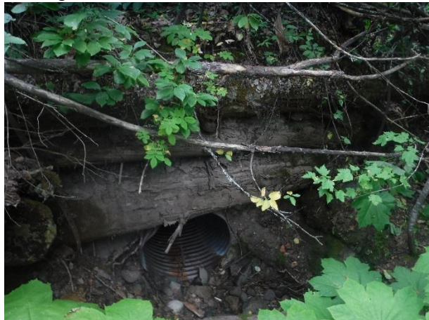
Photo 30. Upstream 900 mm culvert at proposed access crossing with log bundle on top.
