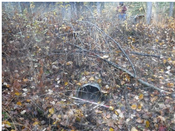
Photo 55: Functional 500 mm culvert (from upstream). Approximately 1 m fill.
