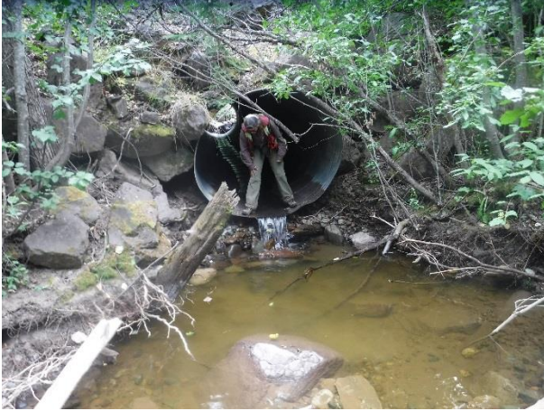
Photo 39. Downstream view of 1800 mm culvert present at the crossing. Nice pool located in foreground with human for scale.
