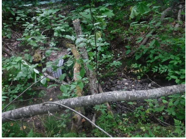
Photo 24. Inlet habitat at 900 mm culvert.
