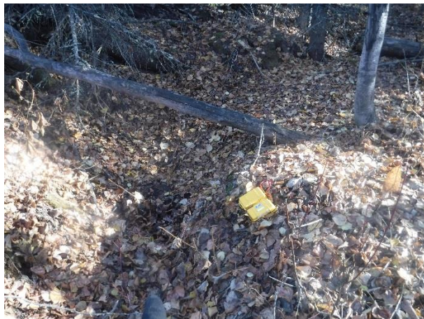
Photo 67: Small draw with no scour located above the road approximately 30 m.
