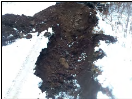
Photo 1: Test pit excavation.
