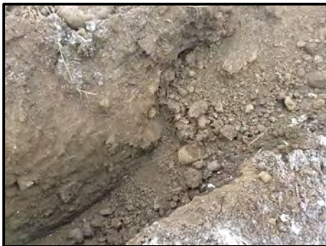
Photo 1: Test pit excavation.
