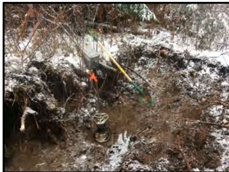
Photo 1: Test pit excavation.
