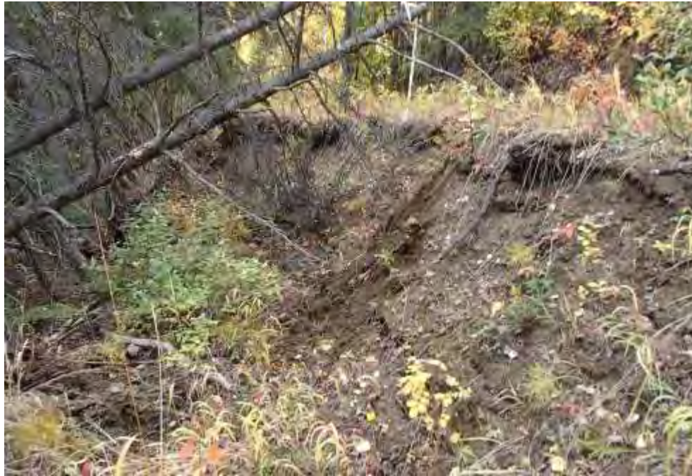
Photo 4: Vertical displacement in the former access road to BVC No 1 Mine.
