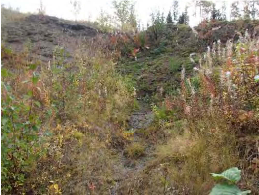
Photo 2: View looking up the slide with seepage zone at the base of the fill.
