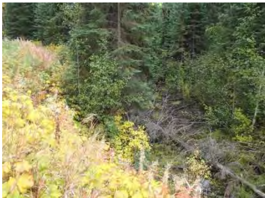
Photo 8: Flood channel below the road that has caused the erosion.
