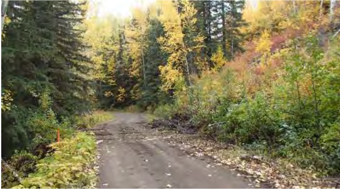
Photo 3: The road near Sta. 11+820 after slide debris had been cleared.
