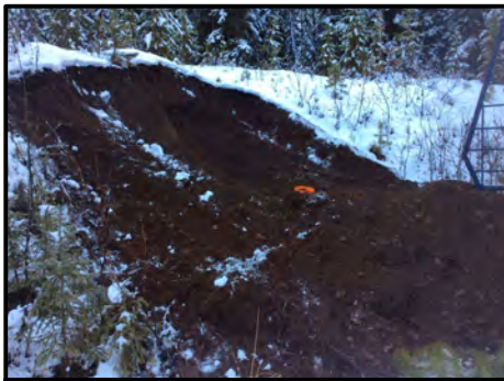
Photo 1: Test pit excavation.
