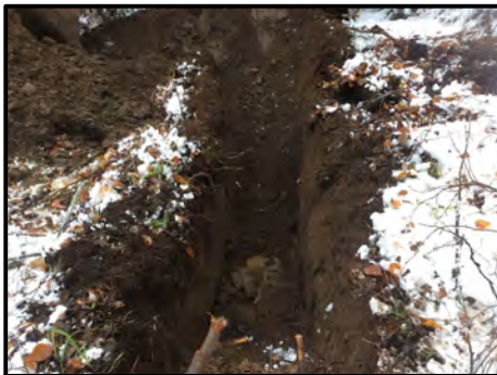
Photo 1: Test pit excavation.
