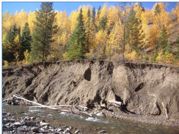
Plate 2-23: Goathorn Creek, undercut streambank exposing mine waste; field site IW240.
