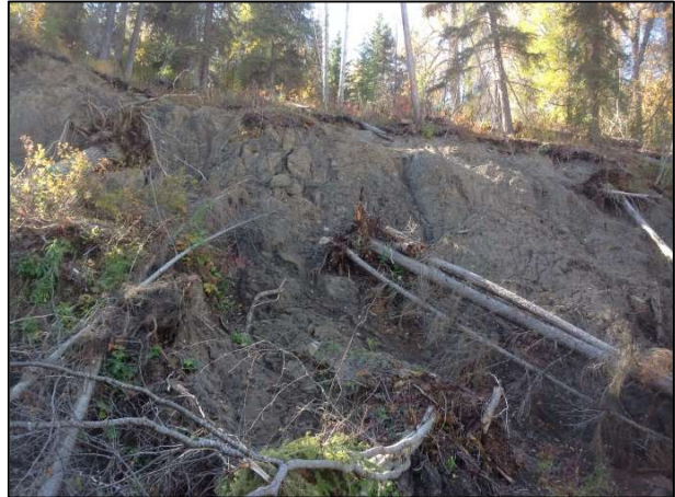
Plate 2-29: Debris slide in till, weathered rock and mine waste along Goathorn Creek; field site IW275.
